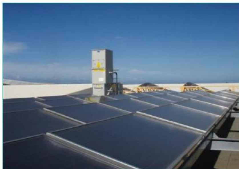
Figure 8: Solar collector field and cooling tower of a small solar cooling system.
