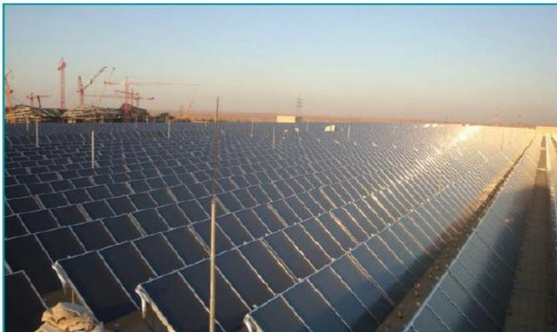
Figure6: The world's largest district heating plant with 25MWth installed capacity (36.000 m 2 ) in Riadh is equipped with European collector technology. (OME report for GSWH-UNEP-UNDP,2012).
